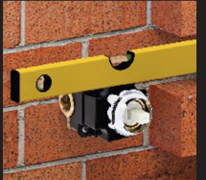
2. Installation of piping to the concealed part.
