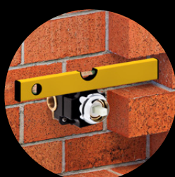
Leveling of the concealed part.
