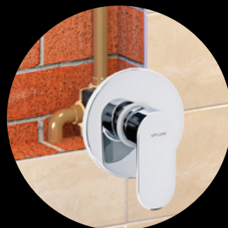
Installation of external components.
